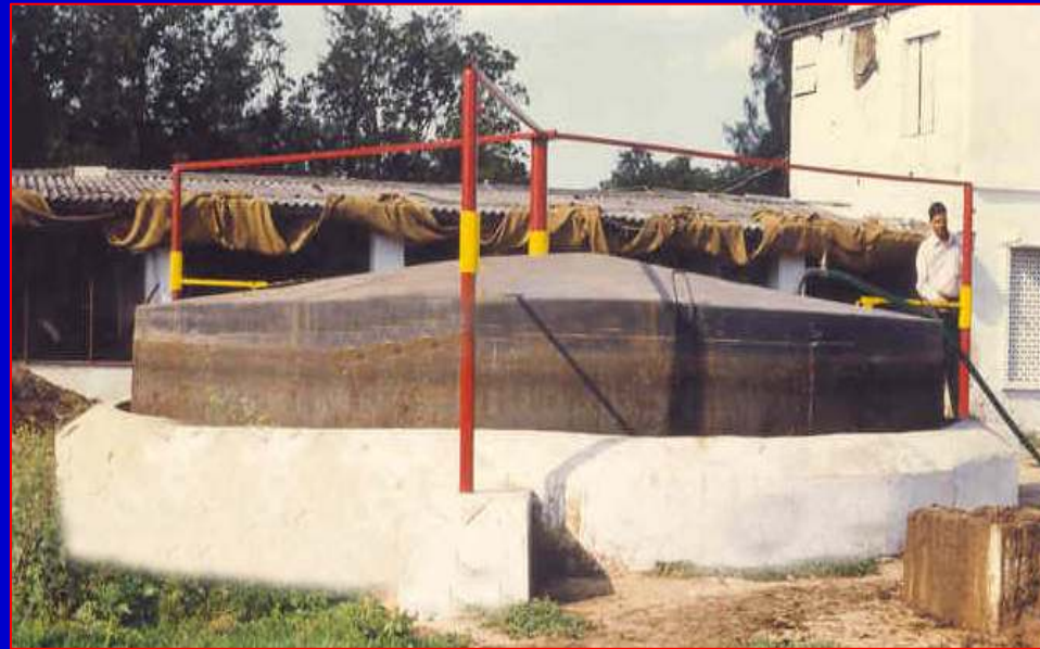
Community biogas plant
