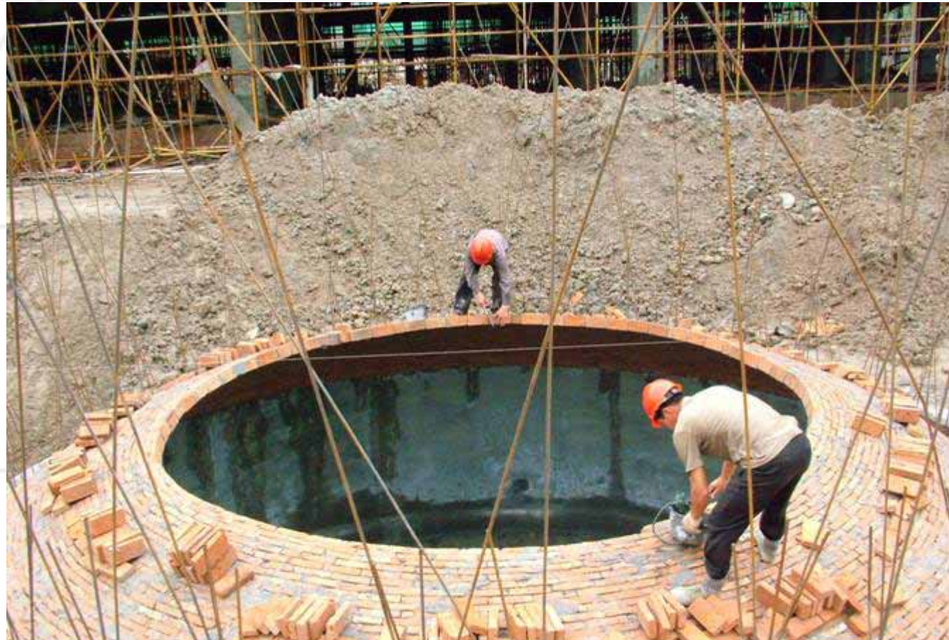
Spherical Digester under construction
