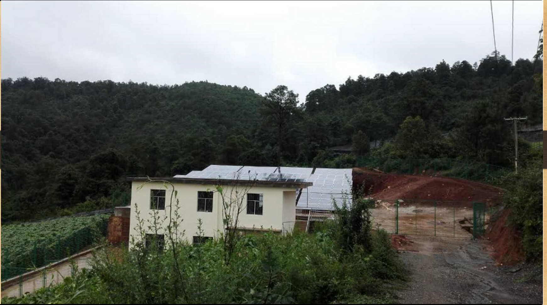
Kong tang qing Solar pumping station
