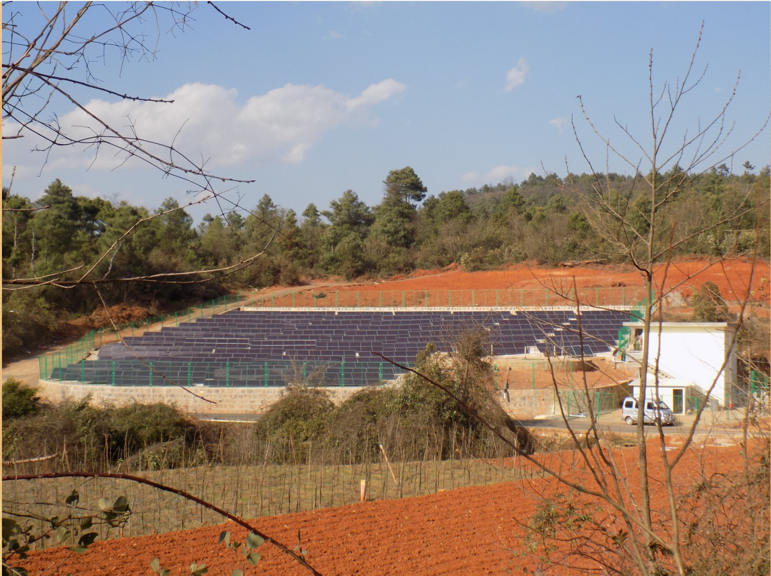
Bo yi Solar pumping station
