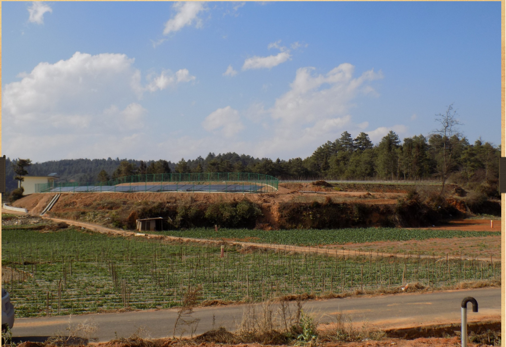
Jiao yuan Solar pumping station
