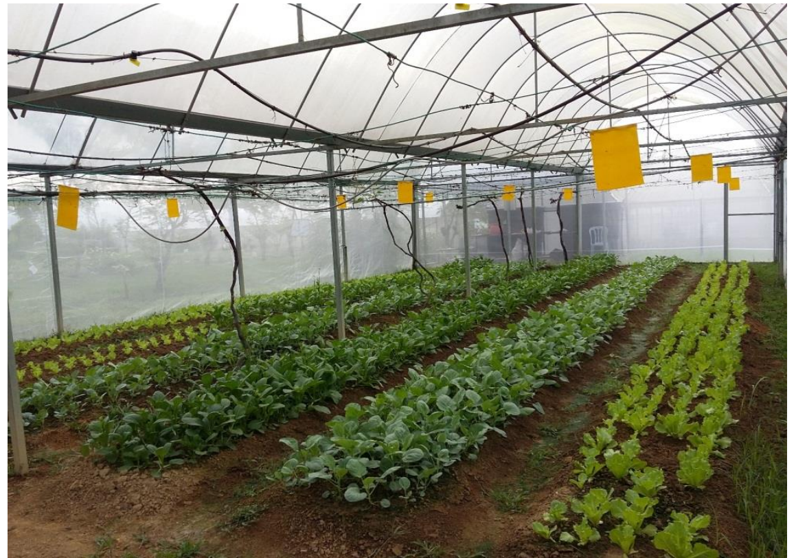
Rainshelter with side netting
